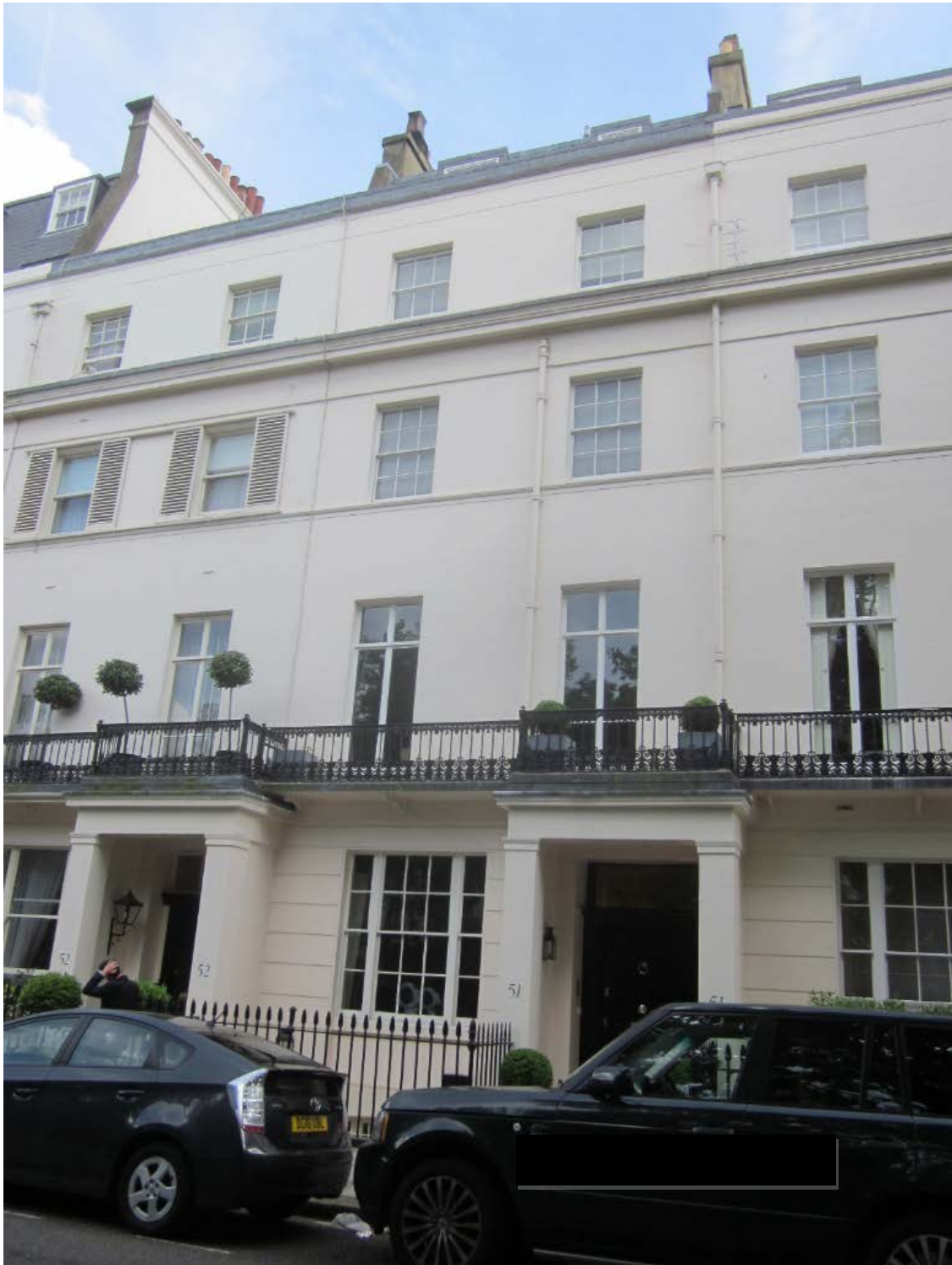
Front elevation of application property
