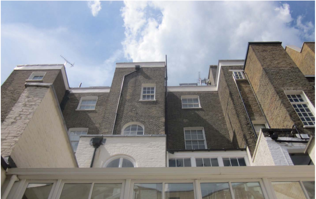
Rear elevation of Nos. 50, 51 (application property) and 52
