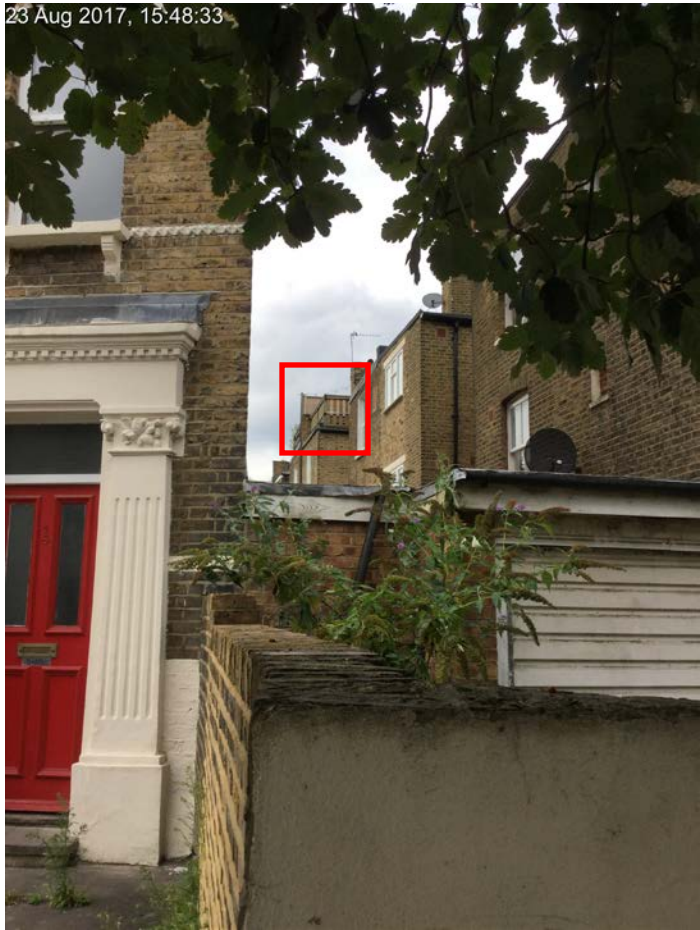
View of fence from Bradiston Road
