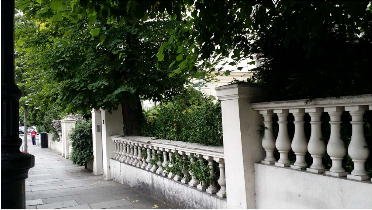
Length of wall to be replaced including two piers to the north.
