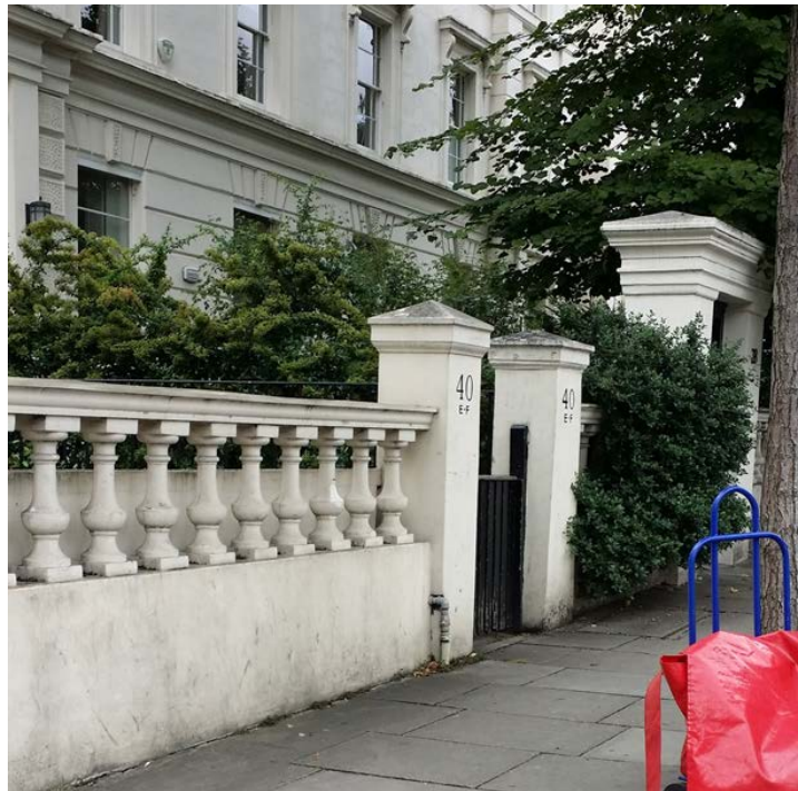
Gate piers to shared access that are to be extended.
